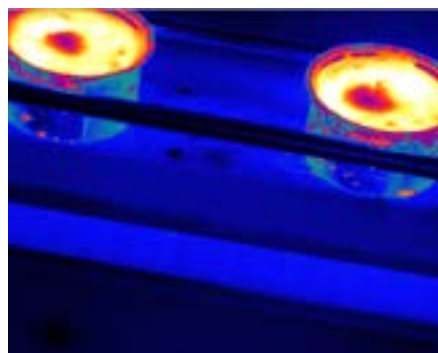
High-speed control and temperature monitoring
